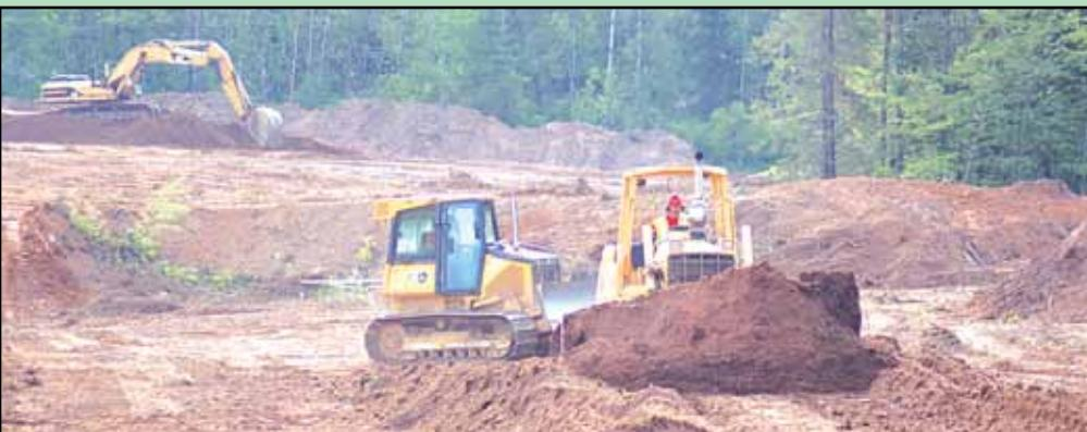
FDL Construction workers are excavating dirt in a field just south of the Sawyer Community Center. The field will be the source of the fill dirt for "west phase" of the Moorhead Road construction project. Photo by Dan Huculak
