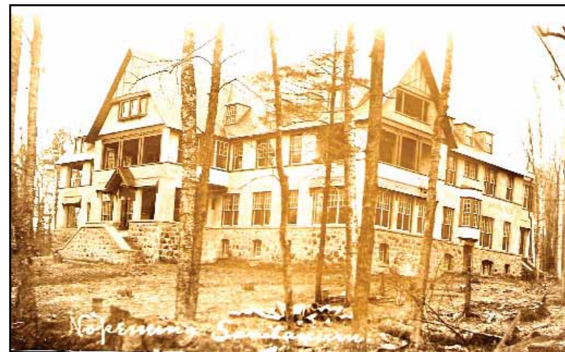
The original Nopeming Sanitarium in 1912. It was known then as the Hart House. Photo courtesy of Christine Carlson.
