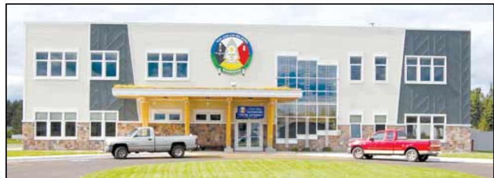
The new Natural Resource and Tribal Court building on University and Big Lake Roads
