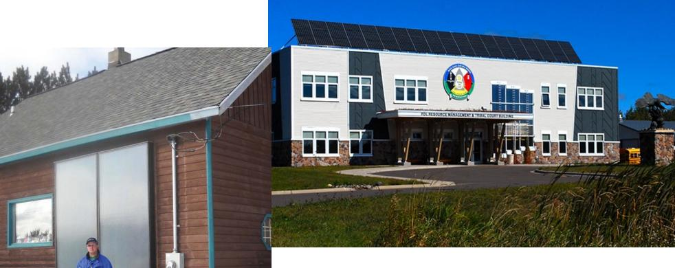
The Tribal Court/ Natural Resource Building is LEED certified which means it was built to use less energy than a standard building. Also to help reduce the carbon footprint of the reservation there is a 12 KW solar panel system on the roof of the building. These solar panels capture energy from the sun and turn it into electricity for the building.
